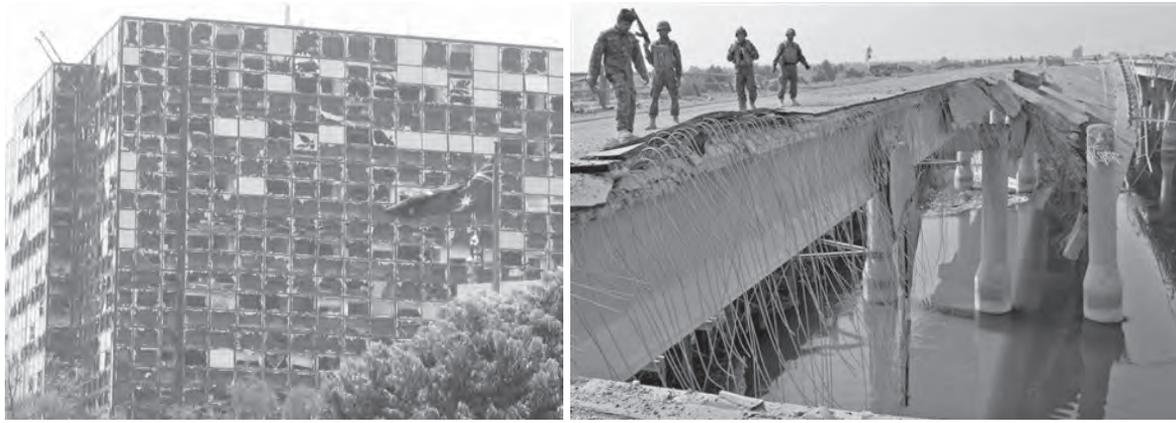
**Figure 1:** Vehicle-borne IED damage to building in Jakarta in 2004 (left) and bridge in Iraq in 2009 (right).
