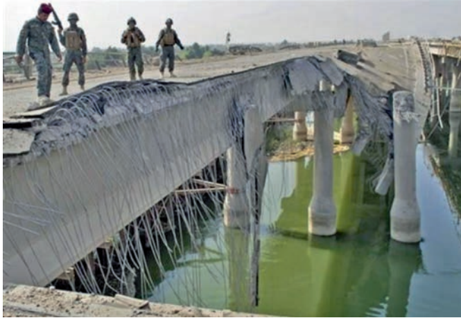
Figure 1. Vehicle Borne Improvised Explosive Device Damage to Bridge in Iraq (47).
