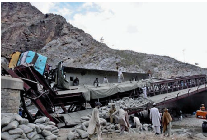
Figure 2. Damage to Bridge in Khyber Pass (66)
