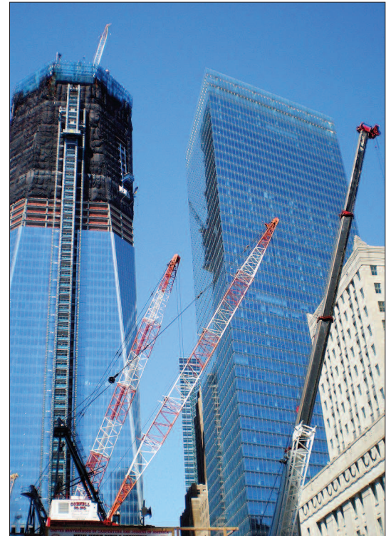
Nearly two-thirds complete, 1 World Trade Center in New York City rises above the site of the twin towers that were destroyed in the Sept. 11, 2001, terrorist attacks. Soaring to a symbolic 1,776 feet, the building, scheduled for completion in 2013, will be the nation's tallest. It is one of five skyscrapers planned for the site.
