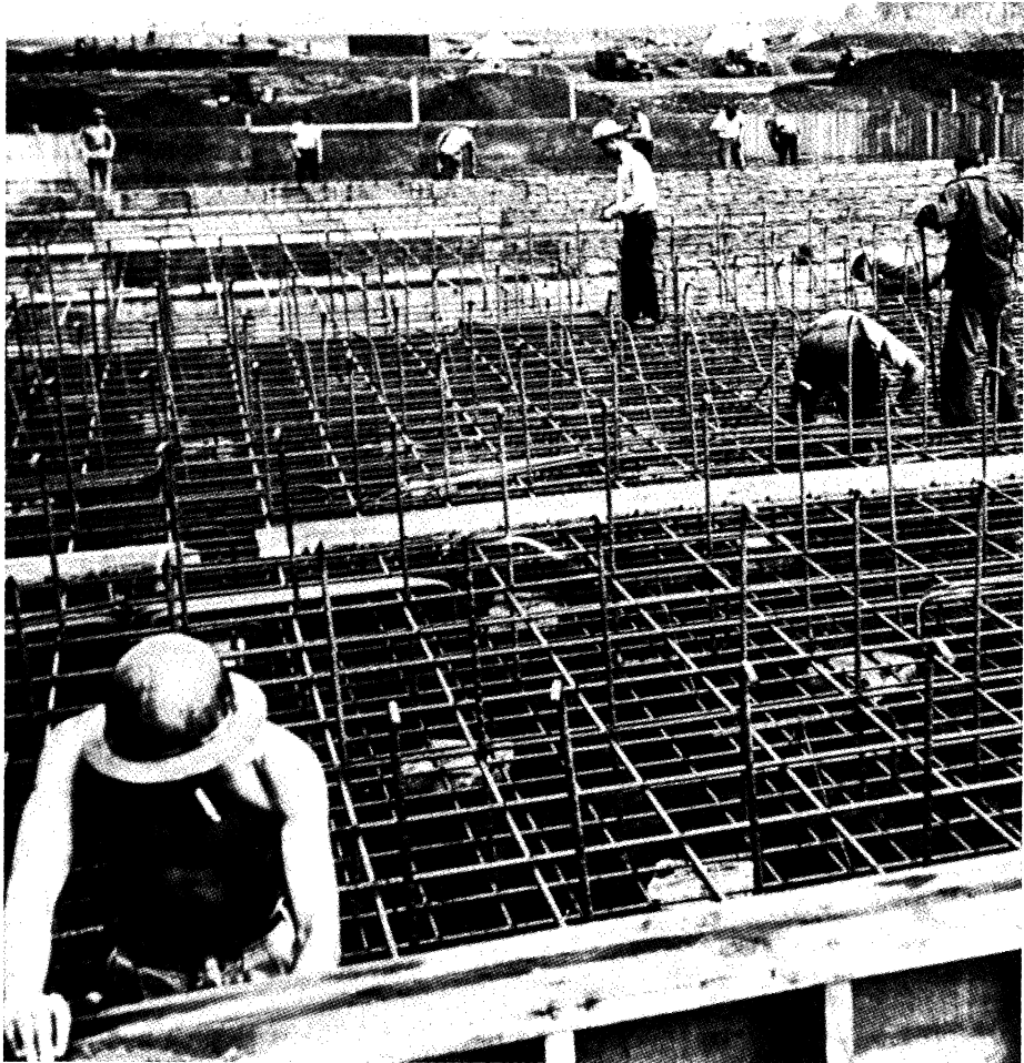
Figure 2. Atypical Pearl Harbor photograph: substantial reconstruction four days after the attack.
